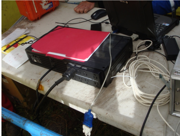
Figure 4-6 UPS Power Supply Backup for Down-hole Probe
