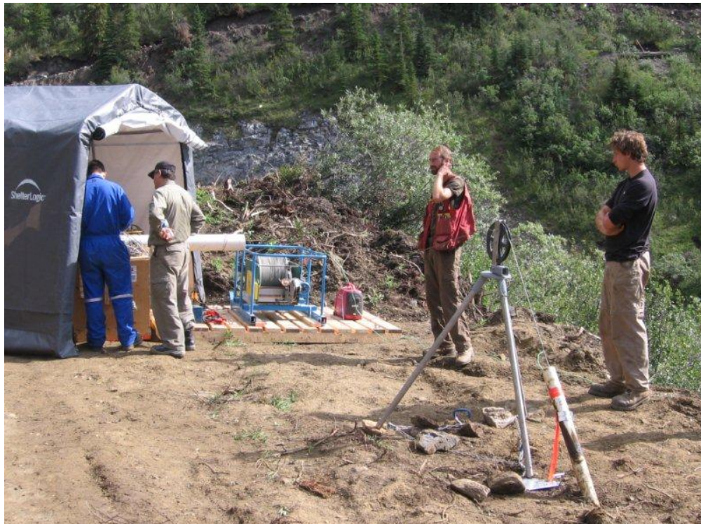
Figure 4-4 Survey Setup with A Plastic Casing and Tripod Mounted Sheave Wheel
